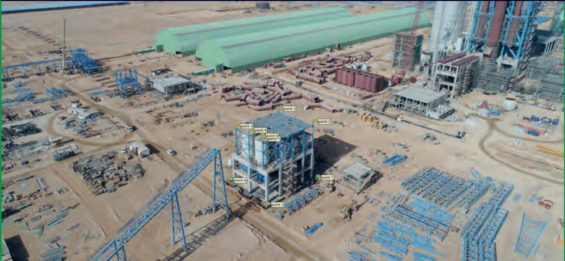
Concrete Plant, Saudi Arabia
